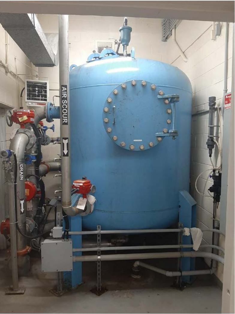
Well 8B/8C Filter Vessel
