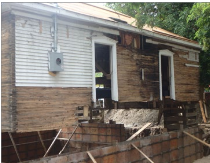
Plank-on-plank wall construction revealed during exploratory work. Note the extent of wood rot exposed when exterior claddings were removed. (City of Markham, 2018)
