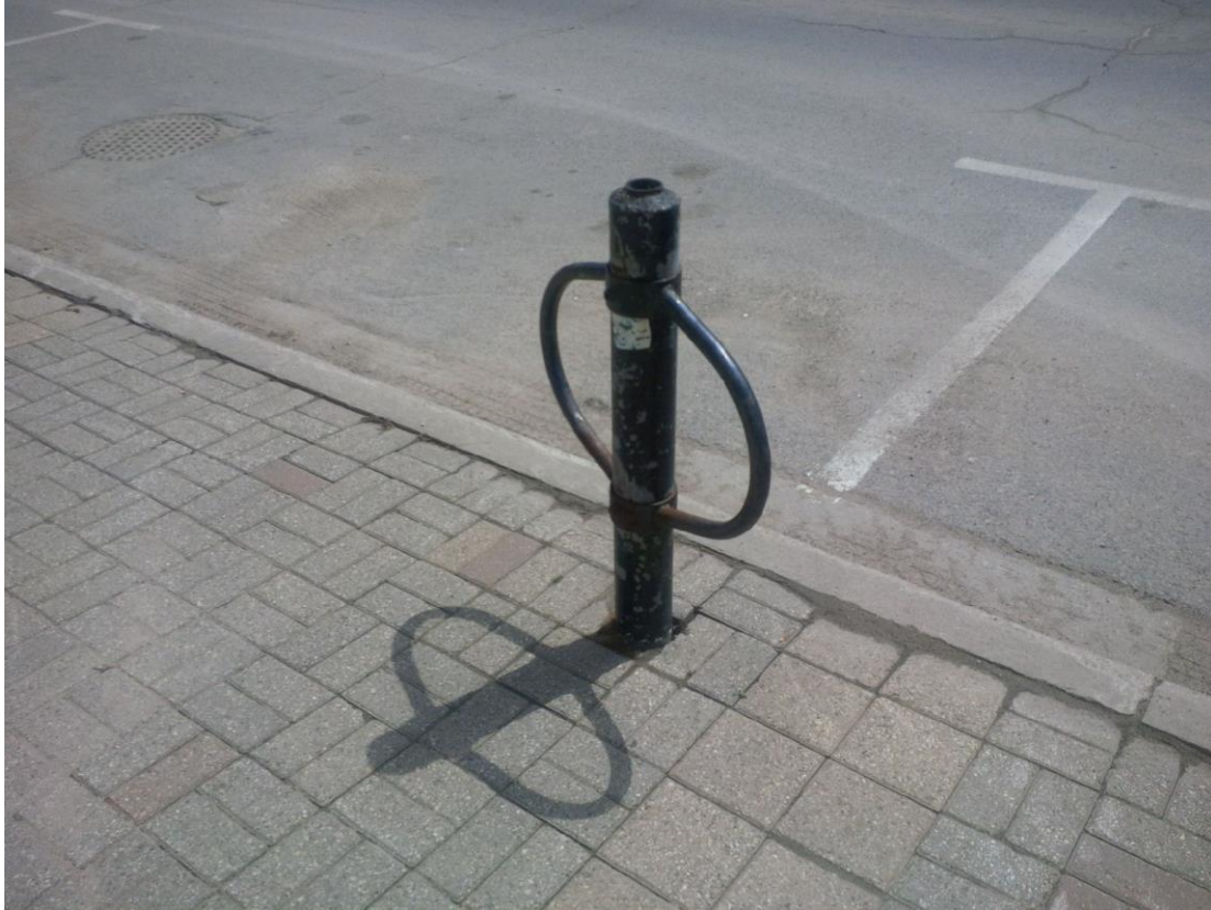
Photo 7 – Parking Metre Posts converted to Bike Racks
