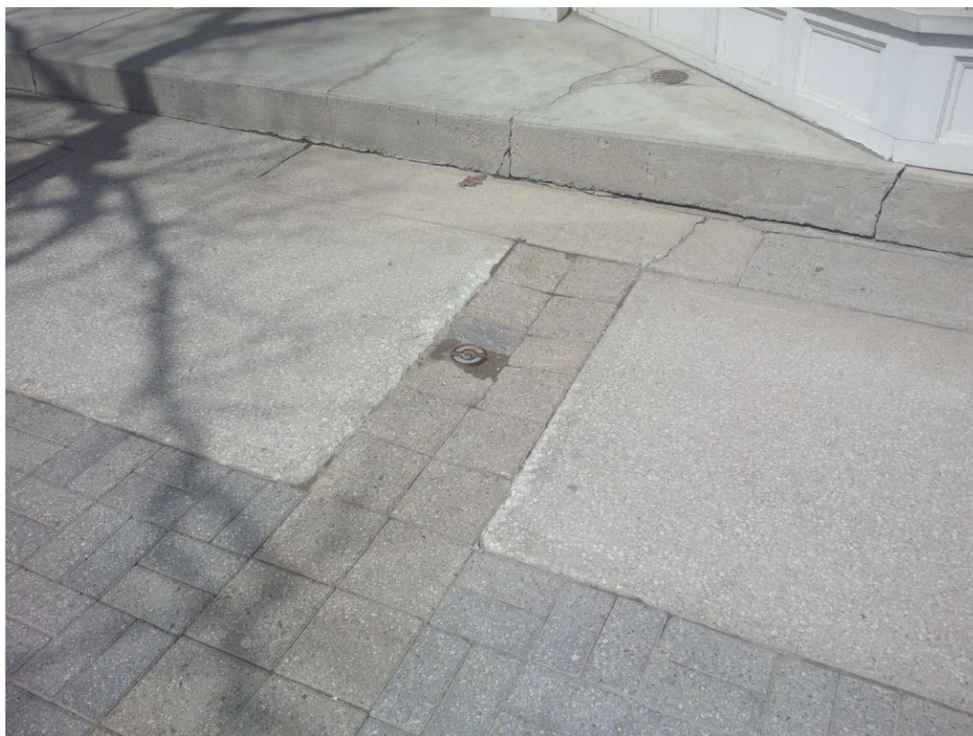
Photo 2 – Settlement in paving stone band and curb stop
