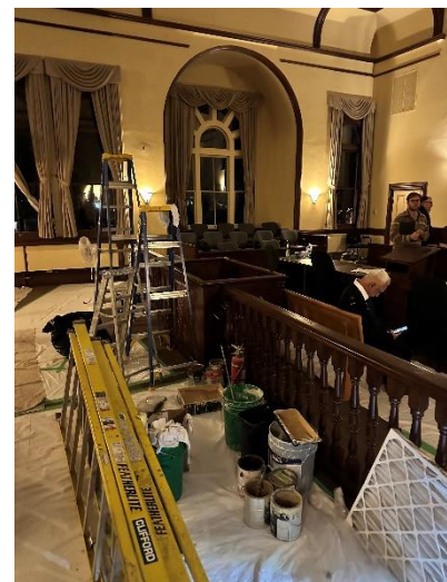
Arched niches at windows, plaster walls, wood trimwork
