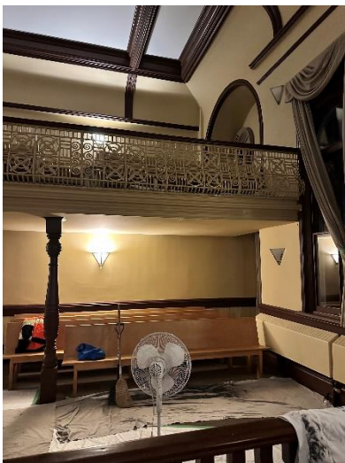
Existing painted iron balustrade with walnut rail at balcony
