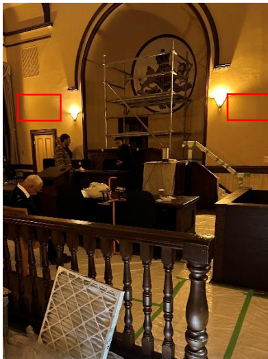
Locations of new wall-mounted display monitors, IR devices and security cameras
