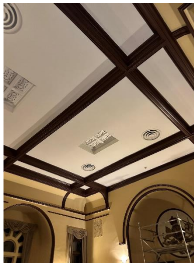
New drywall ceilings with existing wood trimwork
