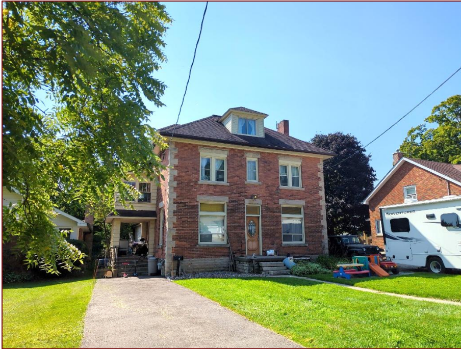
Image 28: East Elevation, 11 York Street
